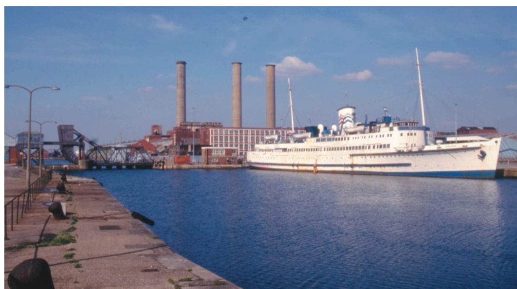
The new canal uses the line of the old central docks, seen here in 1989. Clarence Dock Power Station is in the background, with one of the bascule bridges which gave access to the river bank. The ship is the Manxman , in use as a club at the time.
