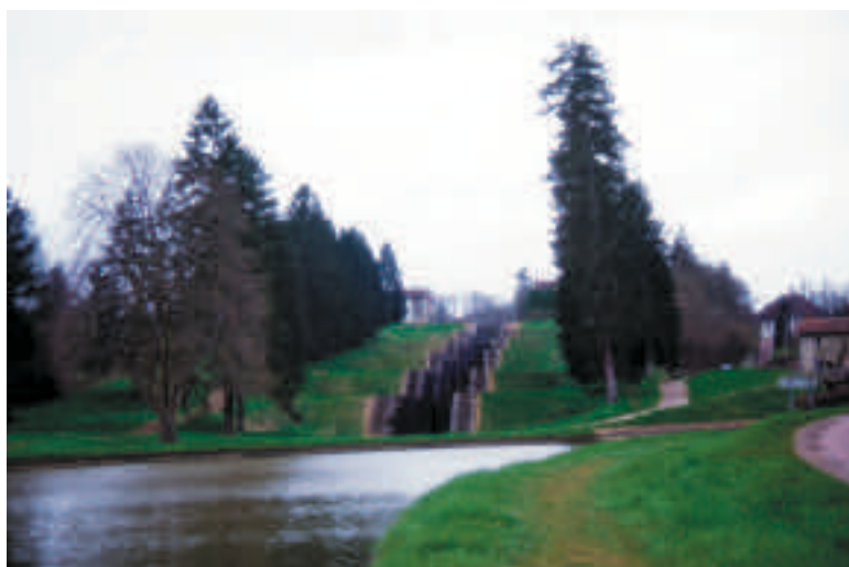
A comparison in the sites of the two most historic riser locks. Above, at Rogny, the locks are placed at right angles to the slope of the hillside. On the right, Bingley can be seen from a distance rising majestically along the side of the valley, a much more dramatic location.
