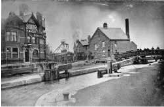
Above: The lock at Plank Lane was moved closer to Wigan because of subsidence, with these photos taken c1910 and c1990. Note that the overbridge in the older photo has now replaced by a lift bridge, and the disappearance of the colliery headstocks.
