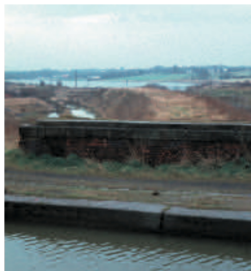
Left: an aerial view in 2001 of the Leeds & Liverpool Canal near Leigh. The now closed and demolished Plank Lane Colliery was centre left, and the large lake, locally called a 'flash', is a result of subsidence. The railway embankment, shown below, is to the right of the canal, just below the abandoned colliery site. The amount of subsidence can be judged by the fact that this railway once crossed the canal by a bridge, whose abutment can be seen in the foreground, next to the towpath. This photo was taken circa 1975, when subsidence was still taking place.
